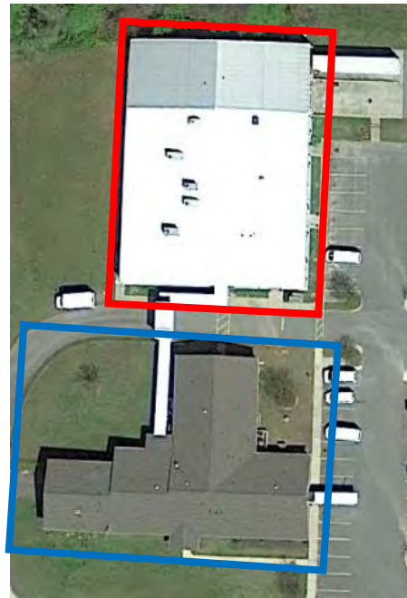
CCDSN Administrative Offices (Blue) and Workshop (Red)
